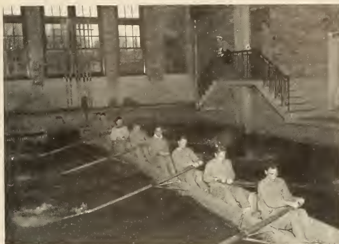
IN THE TANK
